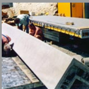
Contenitore per acqua potabile a Schlüsselfeld, 1992
