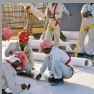
Al Garhoud Bridge Dubai (AE), 2007
