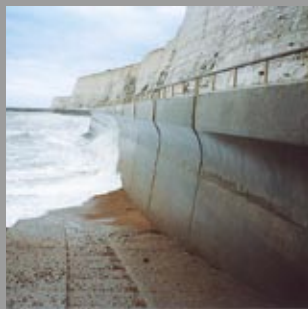
Seawall Brighton (UK), 1992
